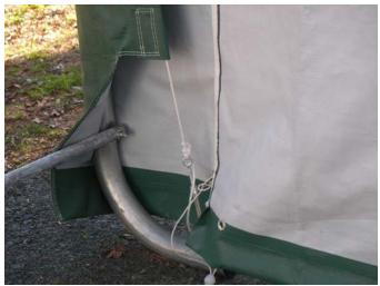
Door Turnbuckle Attached to Base Foot
