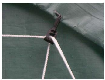
Roller installs on outside rope channel of door
