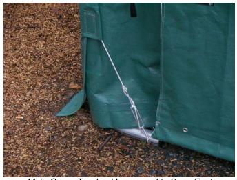
Main Cover Turnbuckle secured to Base Foot
