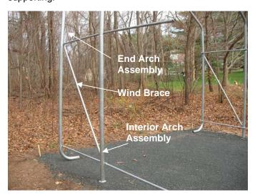
Begin the Top Ridge Cross Rail by placing a #5 Cross Rail <u>underneath</u> the End Arch Top Crest Tube. Secure the Cross Rail loosely with a 3" Carriage Bolt with washer and nut facing the interior of the unit. Male End of next Cross Rail fits into Female end of cross rail. Cross Rails are built by placing rails into each other on the same carriage bolt.
