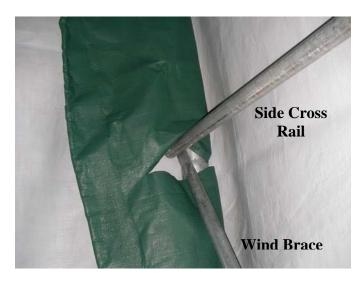
When putting on the doors, adjust the length to make certain the doors do not drape onto the ground. Adjust door length by pulling more or less fabric over end arch. If pulling them up puts too much stress on the slit where it goes over the wind brace, use a sharp knife to cut slit another inch or two to relieve it. The PE fabric is rip-stop weave, and can easily be cut to relieve stress at the frame members.
