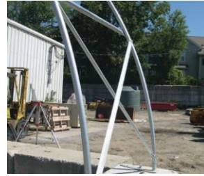
Structural windbrace oneachcorner
